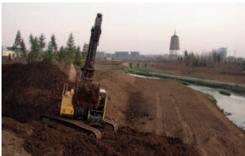
The construction of the Baita Park in Shenyang, China.
