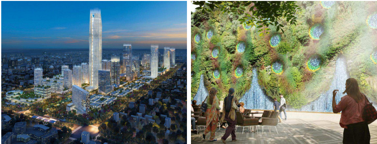
The 150 acre mixed use development at Noida City Centre, Delhi, incorporating a smart and connected cities programme with IBM
